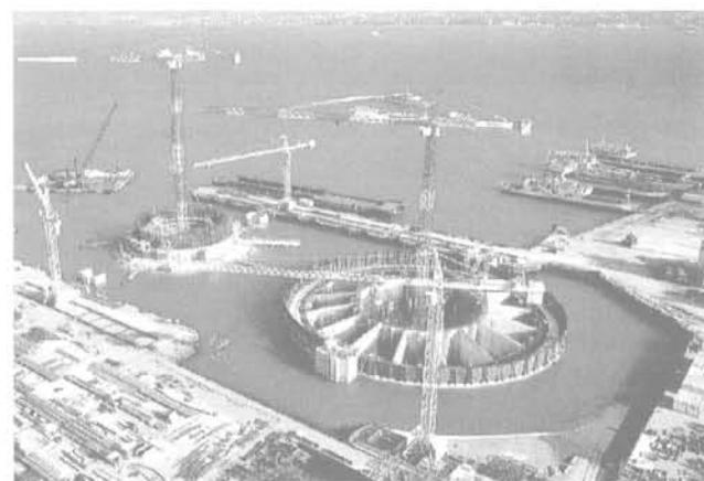
(b) Construction des piles en cale sèche Construction of the concrete footing in the wet dock
